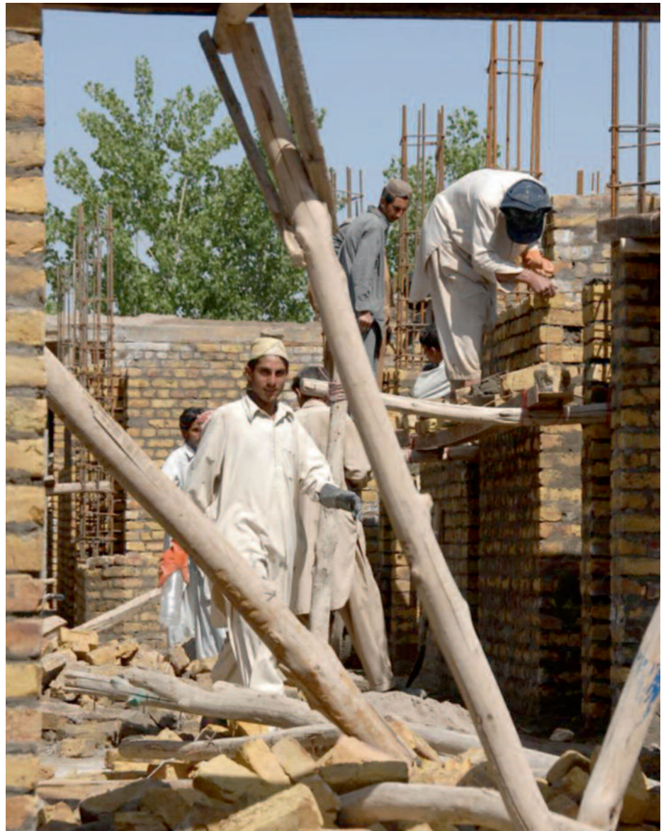
A local contractor constructing a Hospital
